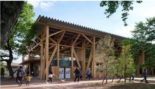
KAKAMIGAHARA PARK BRIDGE
